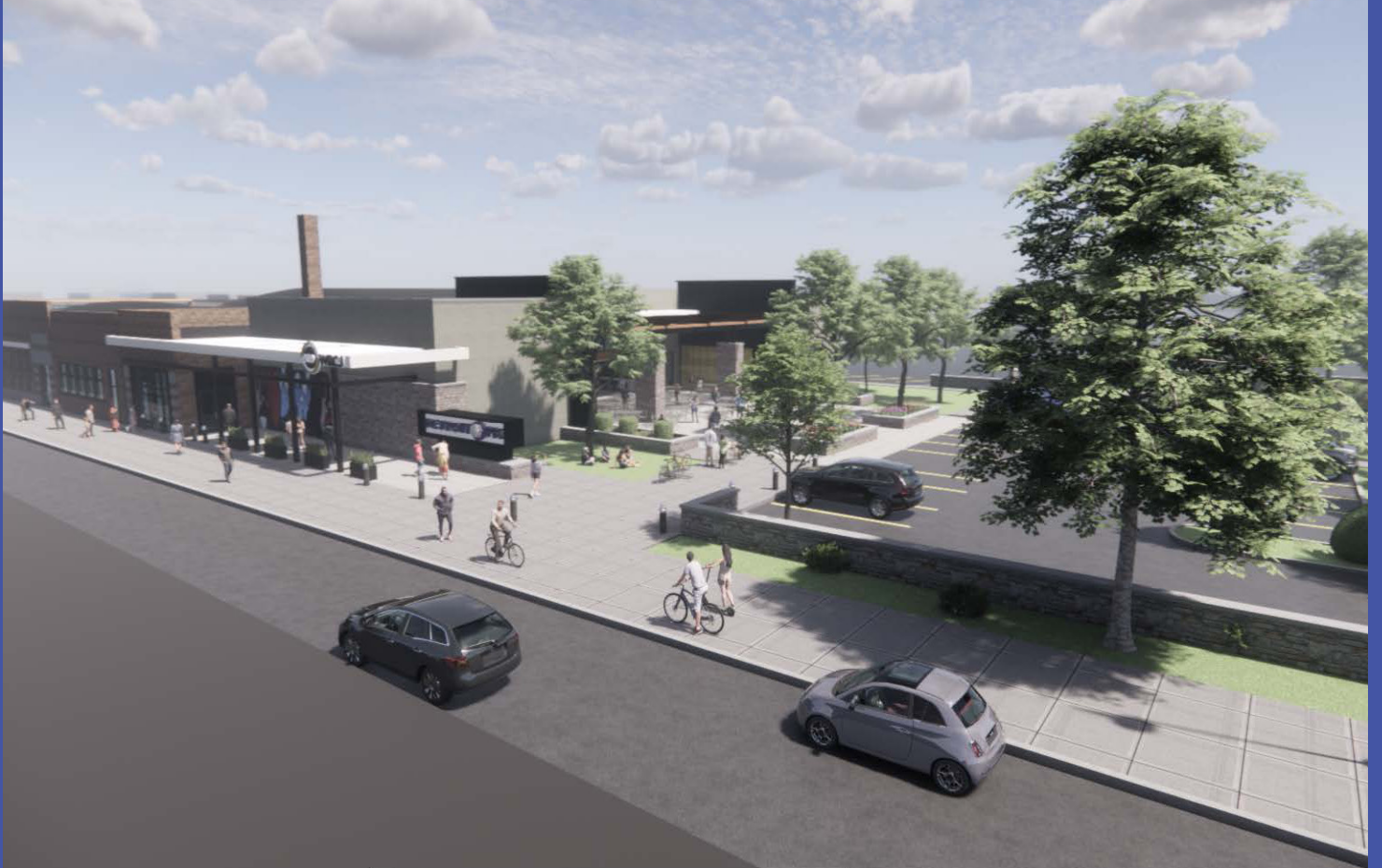
The Detroit Public Media Campus will feature 50,000 square feet of gathering space and over 110 parking spots.
